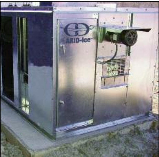
Outdoor slab installation rated at 3,000 SCFM.
