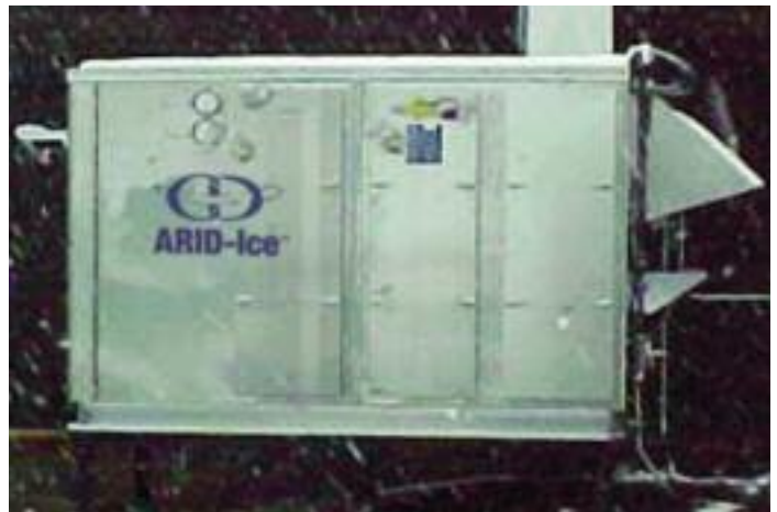
Curbside installation rated at 5,500 SCFM
