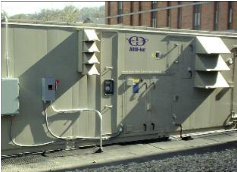
Rooftop installation rated at 15,000 SCFM.
